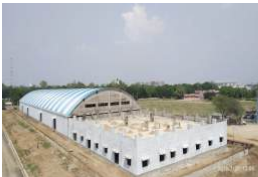
Shed at Sabarmati store depot (under construction)
