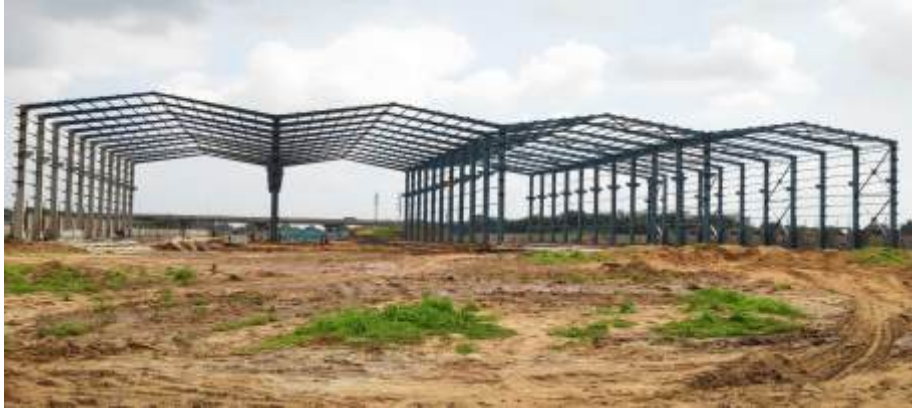
CPOH main shed, Vatva (under construction)
