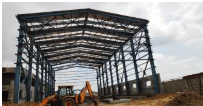
DMC main shed, Vatva (under construction)
